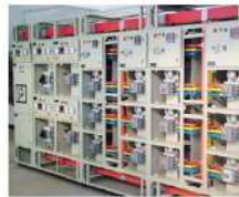
Motor Control Centre Panels
